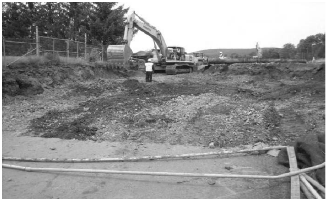
Delaware Street Excavation (Inside the Perimeter Fence)
