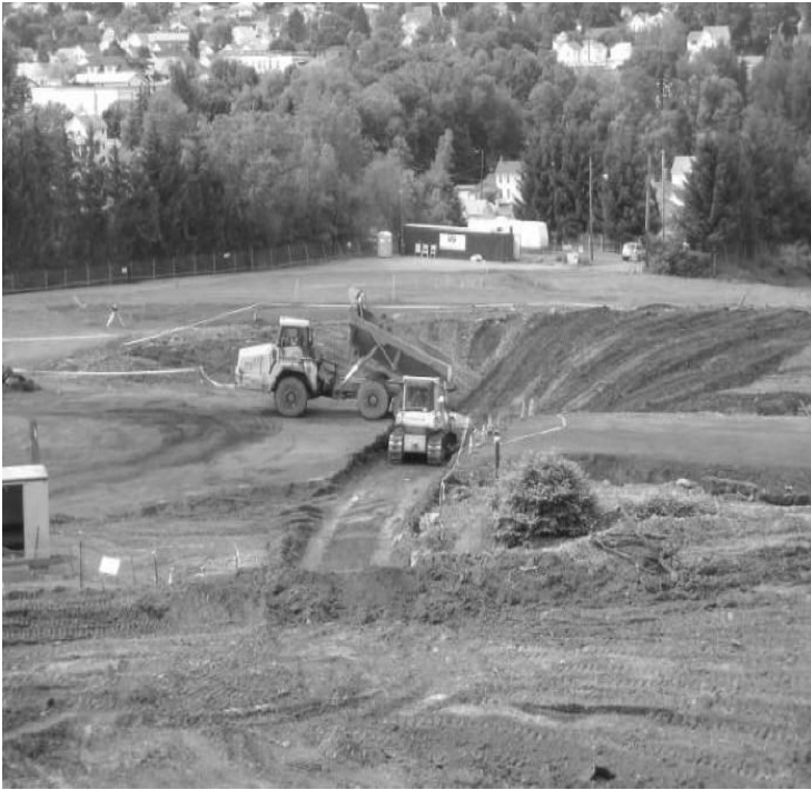
Placement of Material in the Containment (Cap) Area
