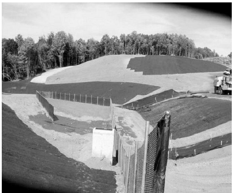
New Sedimentation Basin
